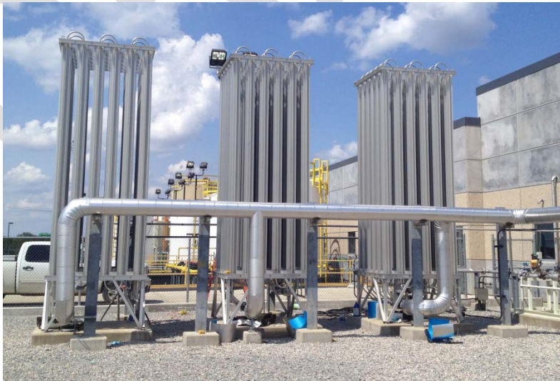
Figure 5-2 Ambient LOX Vaporizers
