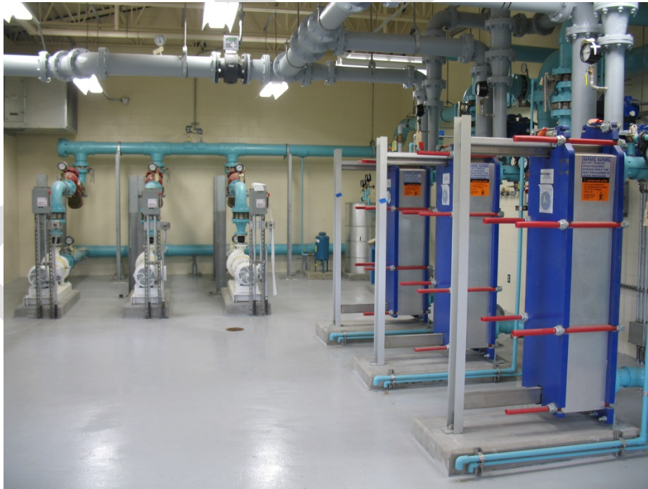
Figure 5-5 Closed Loop Cooling Water System
